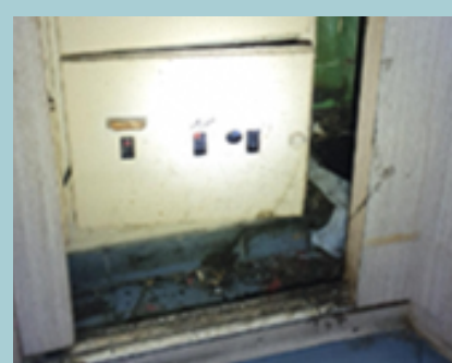
Crevices of wall
